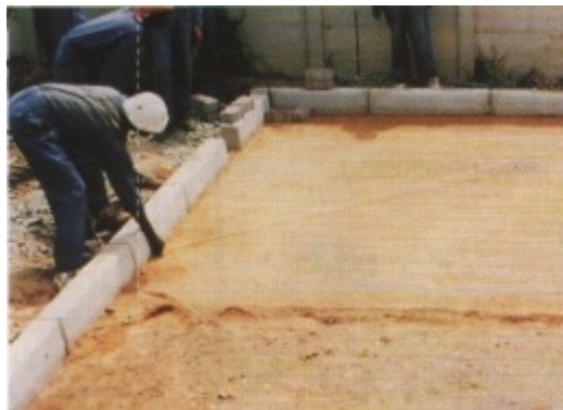
Edge restraints installed before laying commences
