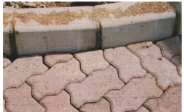
Cutting blocks at edge restraints
